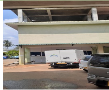
Proposed construction site at the second floor of the building
